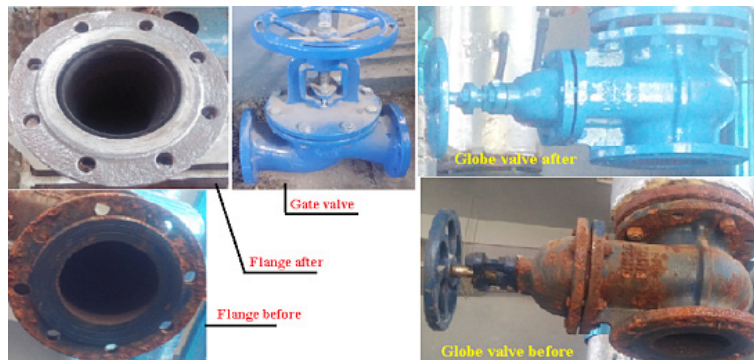
Fig. 6: Accessories for water line before and after repairs
