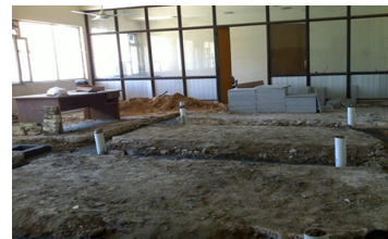
Fig. 4: New four-inch sewage pipes and plumbing were installed
