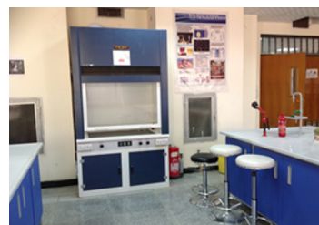
Fig. 8: Fume Cupboards are delivered at each bench if fumed substances are used in a laboratory investigation
