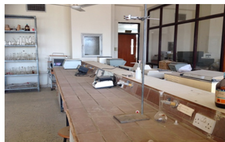
Fig. 2: Old lab benches with deteriorating benchtop surfaces
